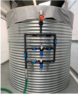
Butyl Aquatabs Tank System (BATS) is a dual dosing unit that provides a direct chlorine feed into Butyl Products Demountable Steel Tanks (Aid/O2/Oxfam models).
